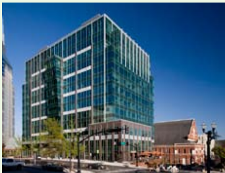
KPMG’s LEED-certified offices in Nashville
